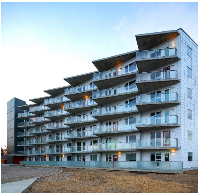
Parkdale ONE. Photo courtesy of GEC Architecture, 2018
